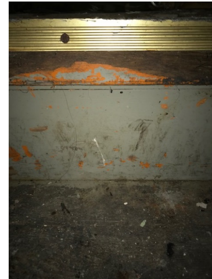
LBP on step riser (stairs to basement).
