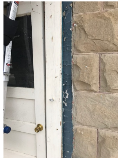
LBP around front door (the green and/or underlying paints).
