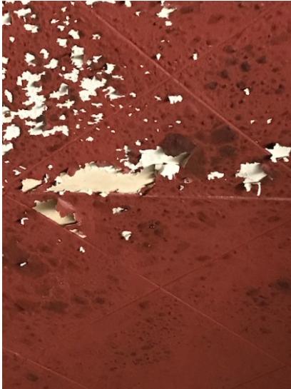
Mold and water damage on ceiling of main level.
